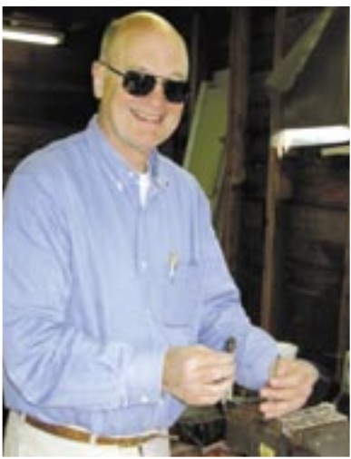
John Doak helping with repairs.
